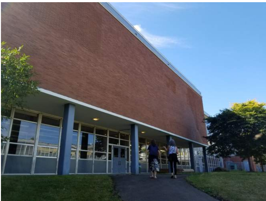
Exterior photo: Music wing cantilever
