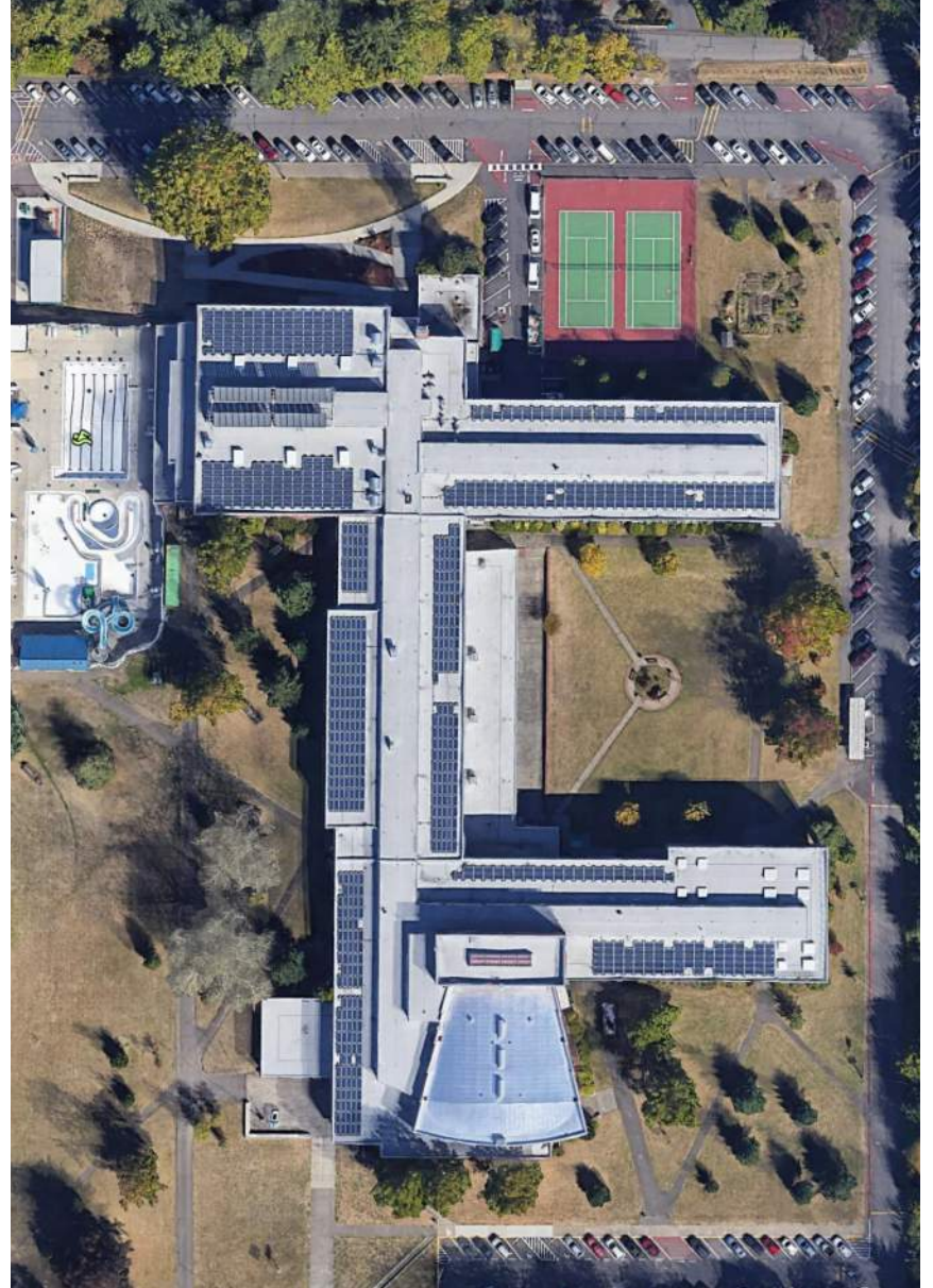
Aerial Google Earth photo: Photovoltaic array
