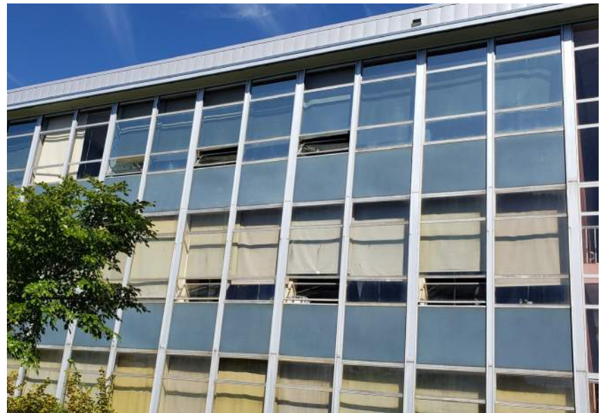
Exterior photo: south-facing classrooms
