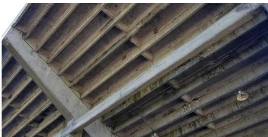
Exterior photo: Underside of stadium seating at track and field
